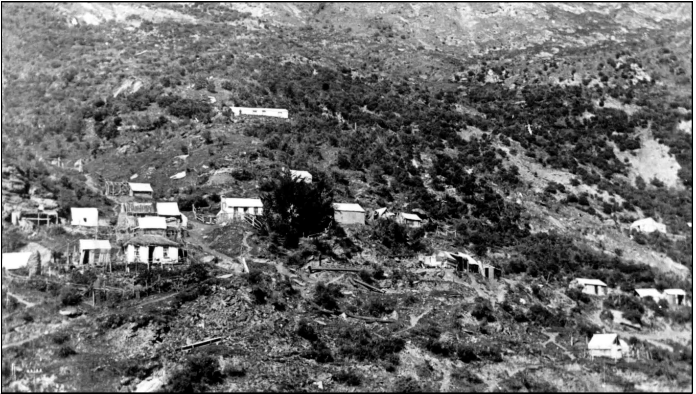
Houses clustered on the hillside at Bullendale
